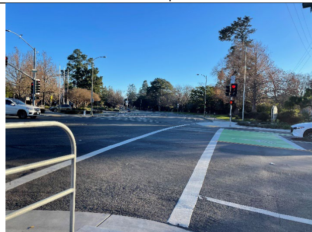
Intersection of Santa Rosa and Sonoma Avenue: Bike box pictured, new ADA compliant ramps
