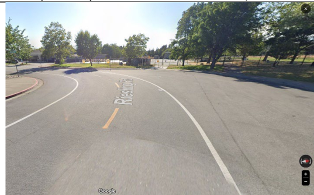
Curve at Riesling/Hartman, approaching Hartman
