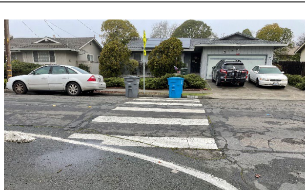
Lance (south side) at Jennings crosswalk – missing ADA ramp
