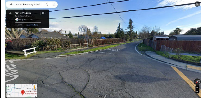
Clover Drive – close up of entrance to roadway with no crosswalk
