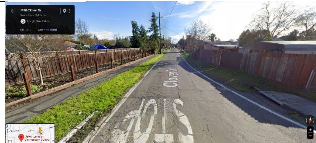
Clover Drive, missing sidewalks, west side
