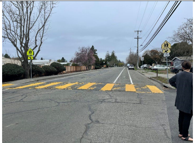
Mismatched signs at crosswalk
