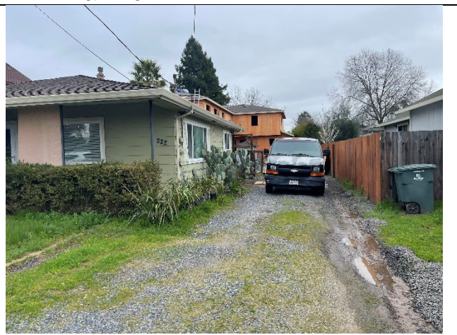
ADU being constructed behind 222 Brittain
