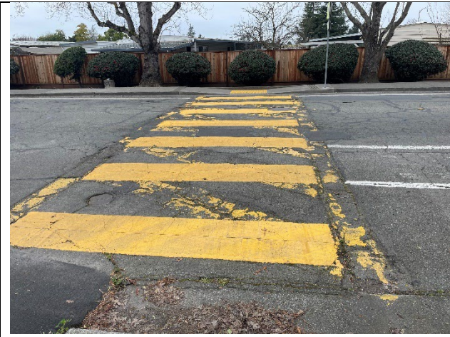
Crosswalk at school driveway/Brittain
