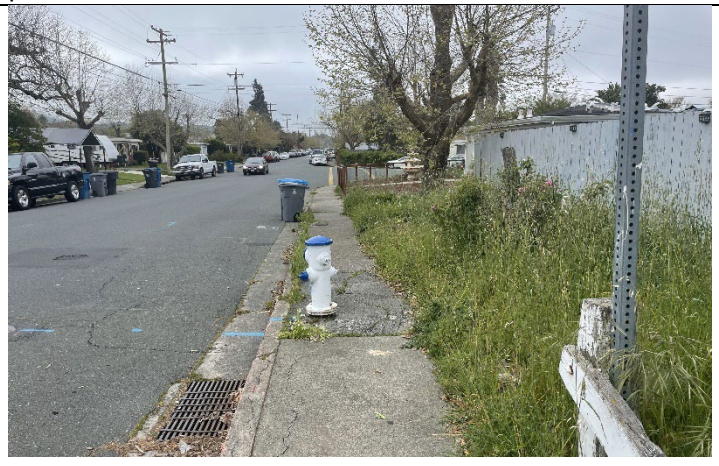
Fire hydrant at Moraga s. of Aston – not ADA compliant
