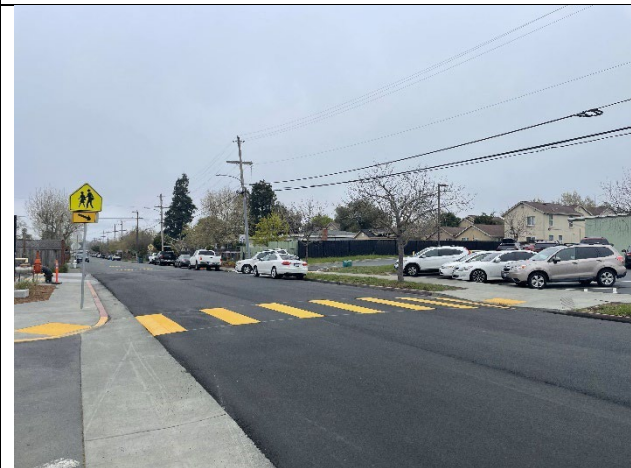
Crosswalk in front of school (signage & pavement markings need improvement)
