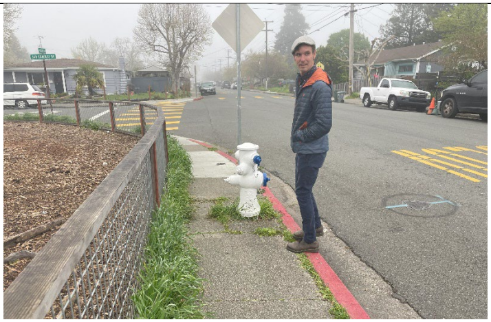
Fire hydrant at Moraga & San Domingo – not ADA compliant
