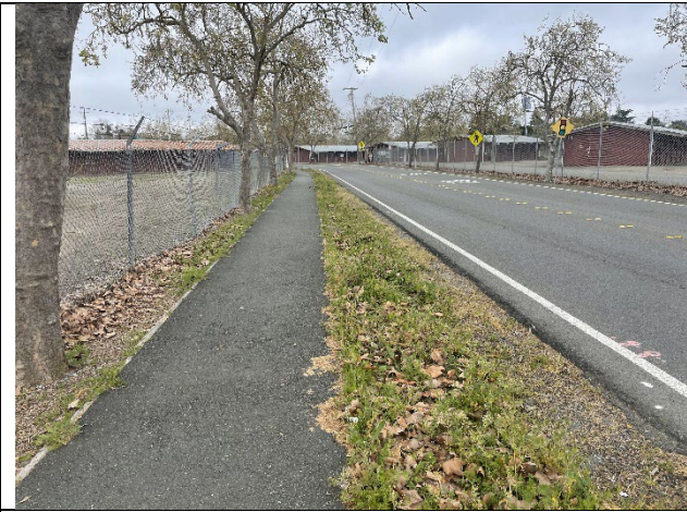
Pathway along s. side of Aston between Moraga & Hendley – consider widening
