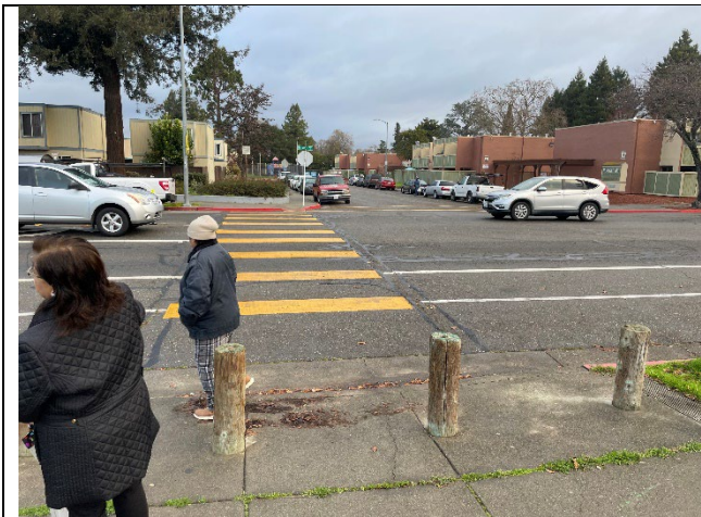
Intersection of Rockwell and W. 9 th – consider RRFB and shortening crossing distance (city)
