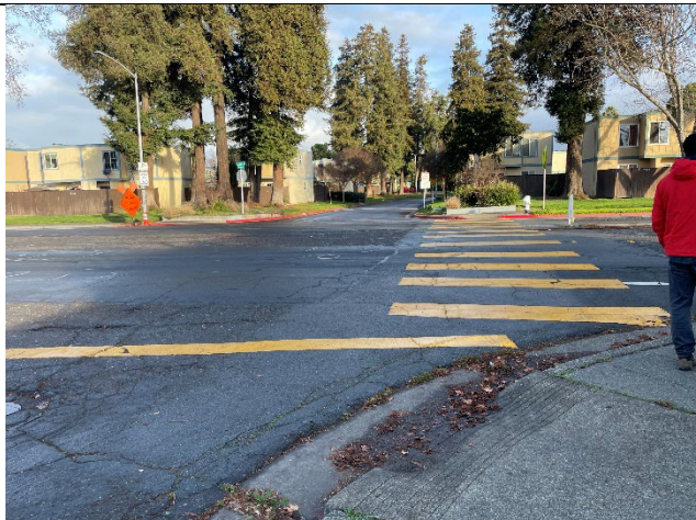
Simpson & W. 9 th (re-install broken crosswalk sign)
