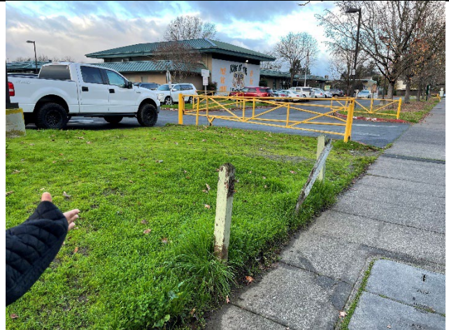
Car drivers hop the sidewalk through this broken barrier to enter school parking lot when gate is closed/park.
