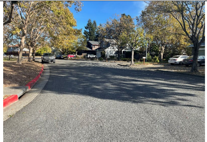
Yarberry Drive is a very wide street
