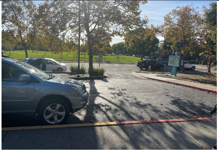
Non-regulation right-turn only sign – replace with regulation sign to enable enforcement
