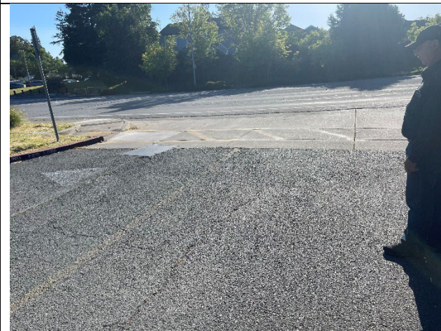
Faded left turn only and right turn only lane markings at school driveway exit (and faded crosswalk)
