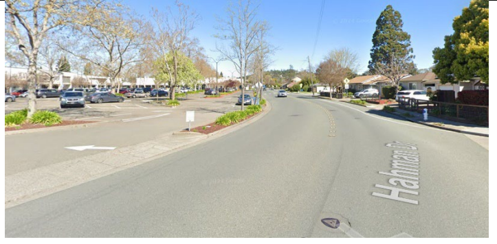
Sidewalk gap continues, students must navigate parking lot
