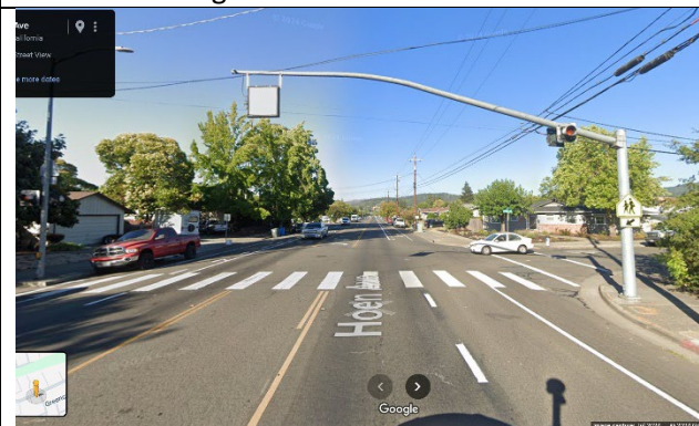
Pedestrian activated flashing beacon at Hoen and east end of Cypress, consider a median or bollards to slow traffic/provide protection for peds.
