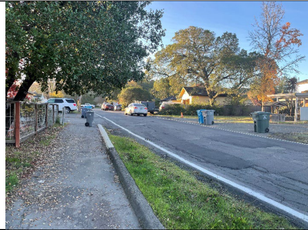
Pathway on east side of Franquette that becomes flooded, overgrown
