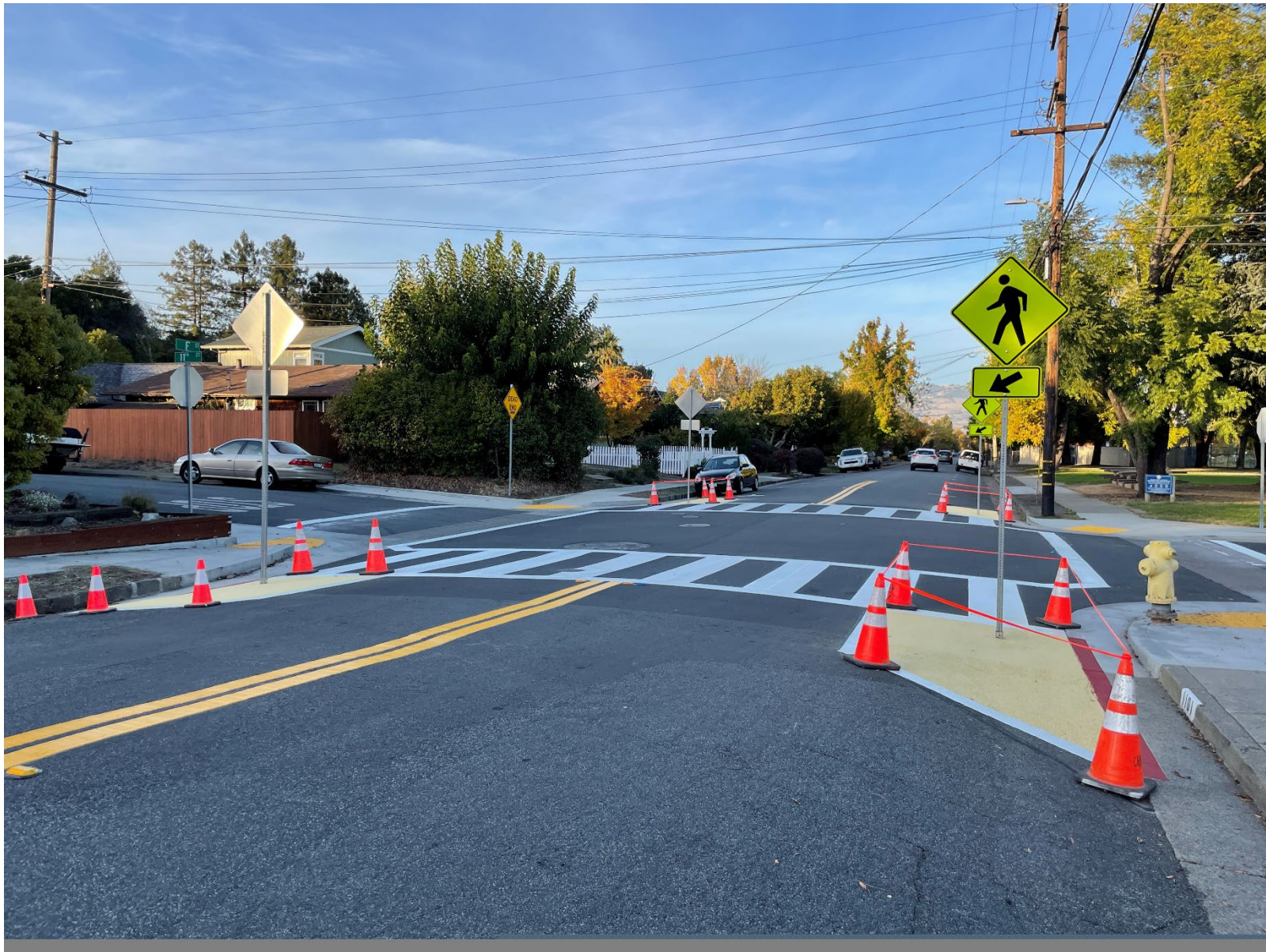
NEW PAINTED CURB EXTENSIONS AT F/11 th
