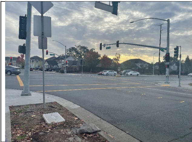
Intersection of Stony Point & Giffen: many safety concerns
