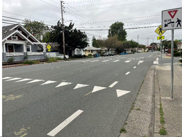
Crossing at Steele Lane & Major Drive (future RRFB?)
