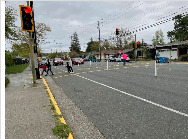
Crossing in front of school – students in “safe zone” inside delineators.
