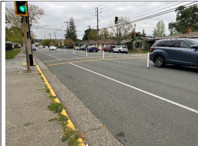
Pilot project in front of school (before drop-off)
