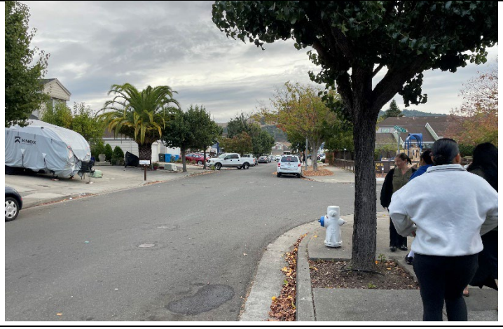
Intersection of Powderhorn and Terrimay – daylight curbs, consider conversion of roadway to class III bicycle facility.
